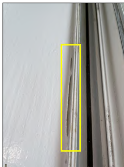
Deteriorated caulk
