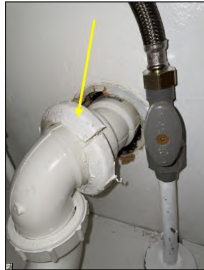
Loose and broken escutcheon
