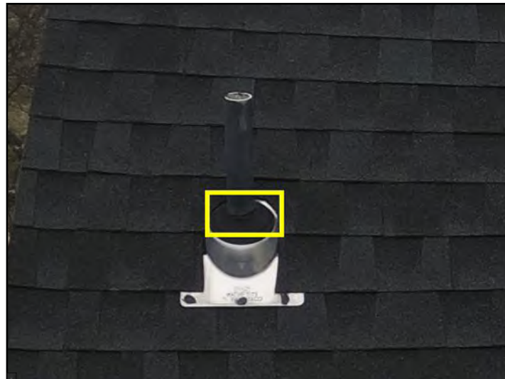
Deteriorated collar
