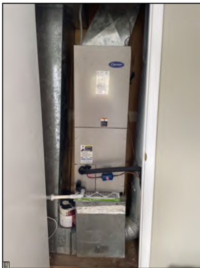
Missing shut off switch
