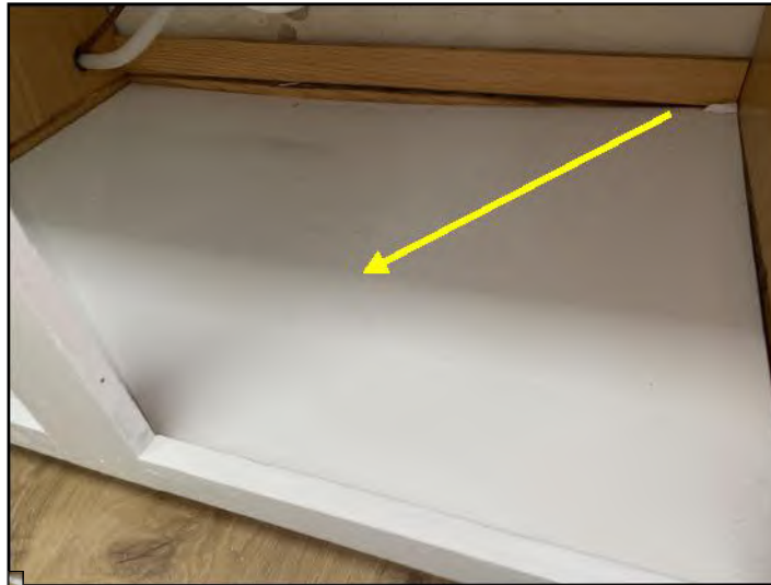
Warped base
