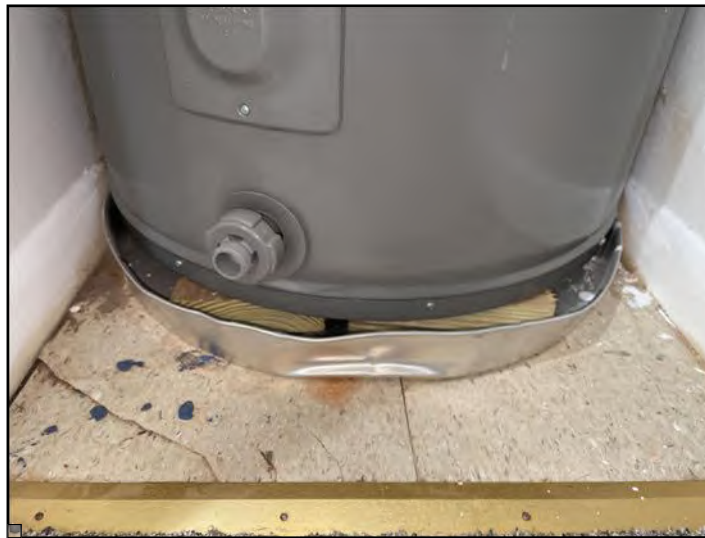
No visible drain on pan
