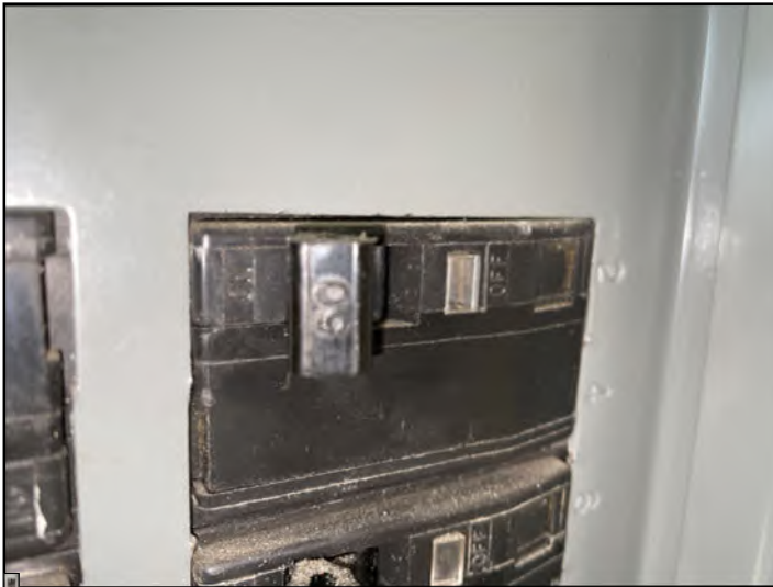
50 amp furnace breaker
