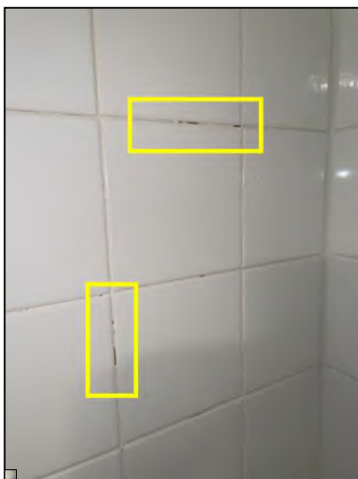
Missing grout
