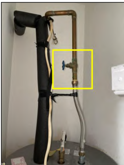
Water shut off valve
