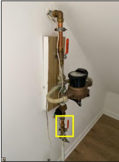
Main water shut off valve
