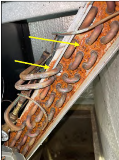
Corrosion
