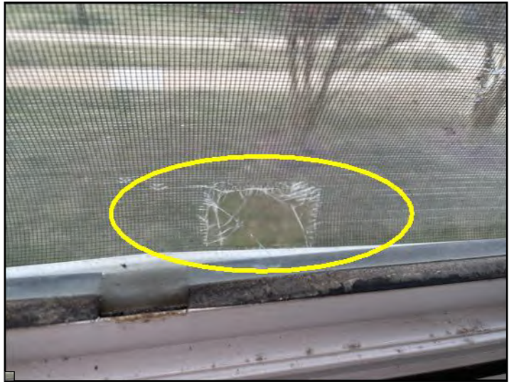
Damaged screen
