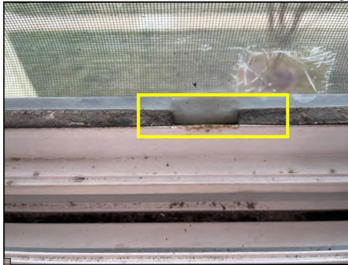
Deteriorated glazing bead
