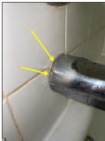
Deteriorated caulk
