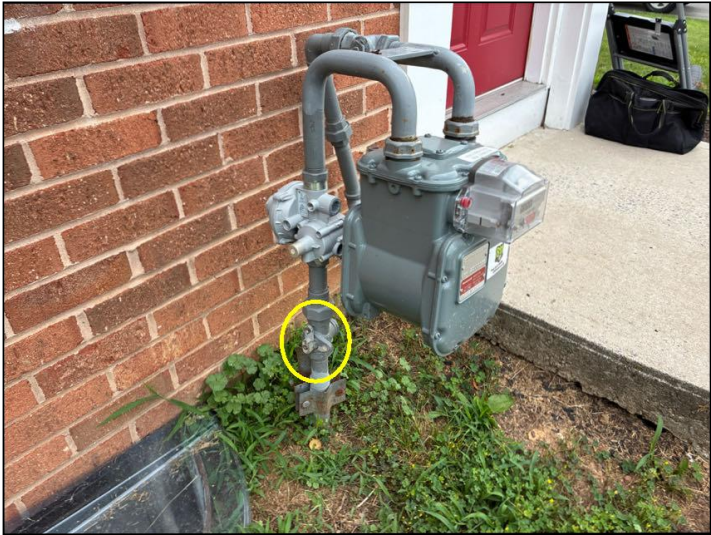
Main gas shut off valve
