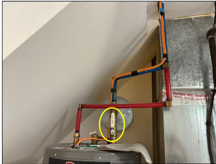
Water shut off valve
