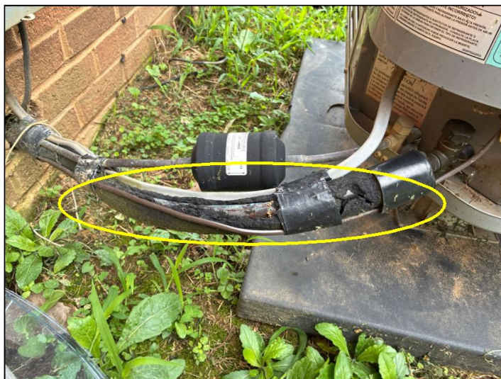
Deteriorated insulation
