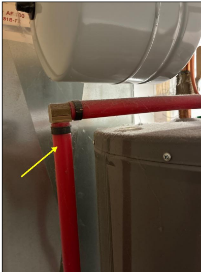
Overflow discharge pipe
