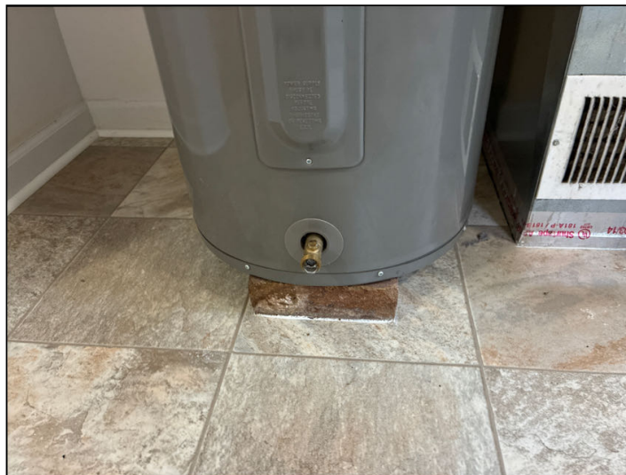
Missing overflow pan and drain
