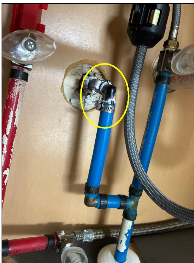
Shut off valve missing
