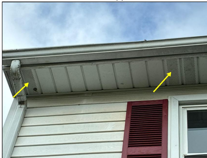
Soffit vents
