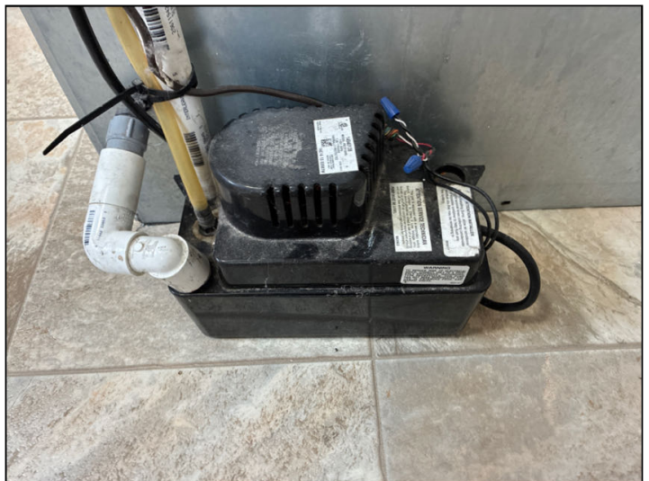
Condensate drain pump
