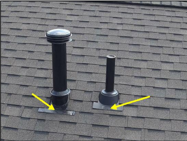
Unsealed fasteners
