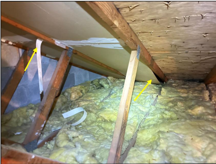
Peeling drywall tape / loose panel
