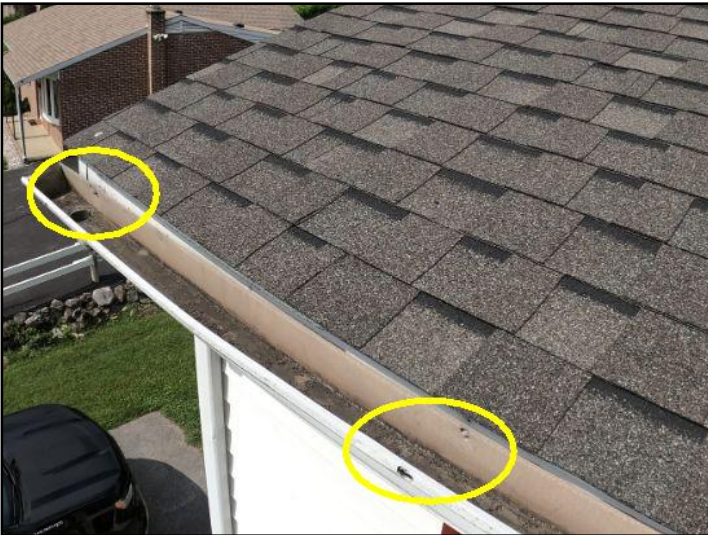
Fasteners missing
