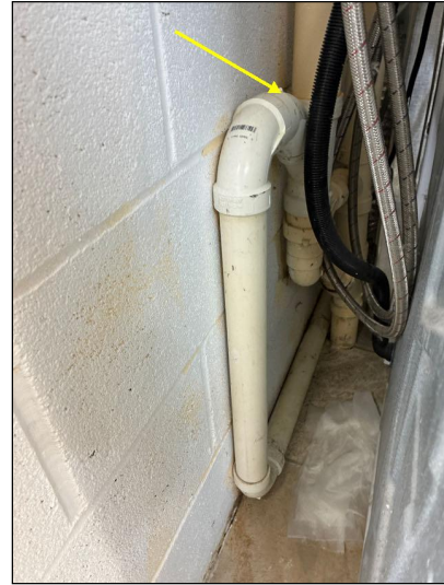
Drained to waste stack
