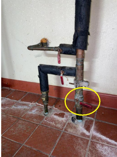
Main water shut off valve
