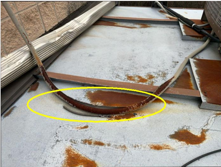
Deteriorated sheathing
