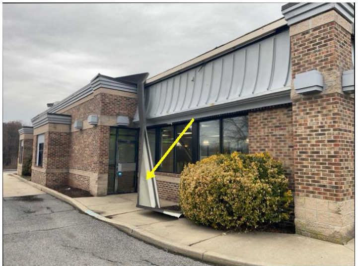
Loose parapet flashing
