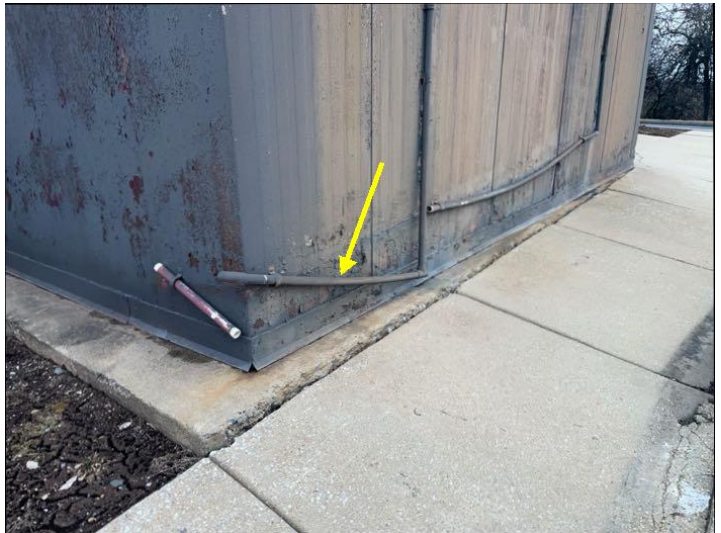
Disconnected drain
