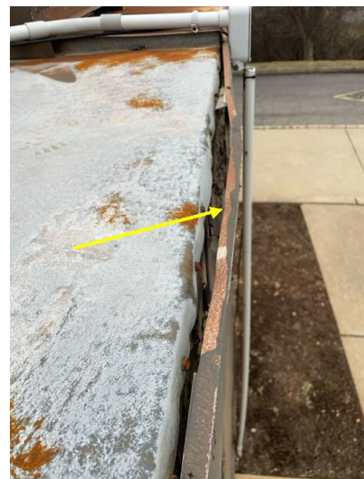
Loose flashing
