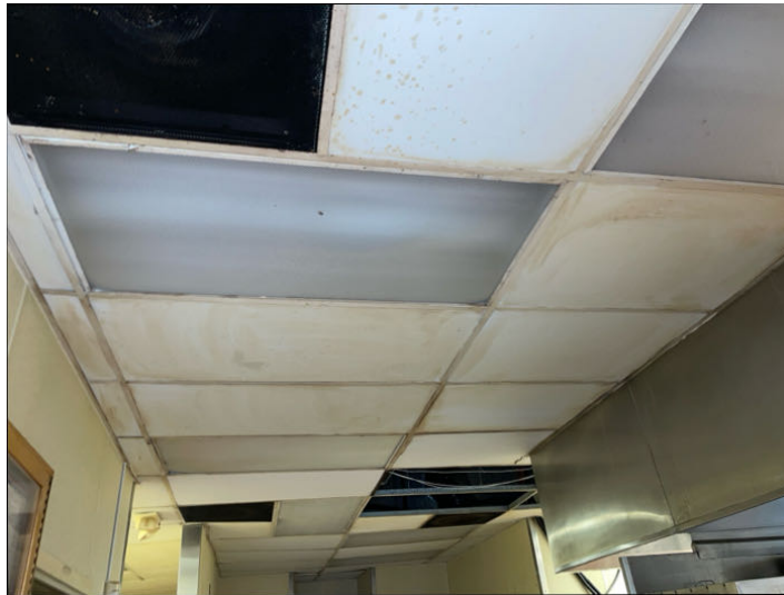
Stained and missing tiles
