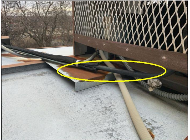
Deteriorated insulation
