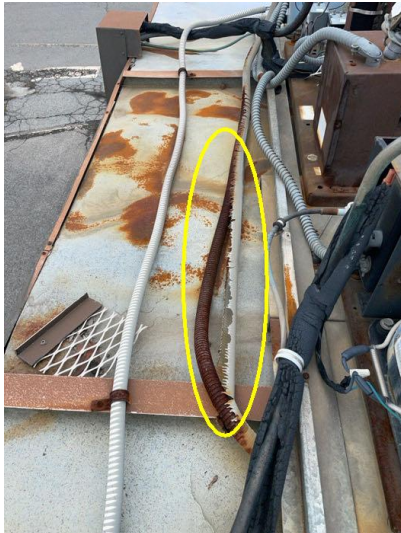
Deteriorated sheathing / corrosion
