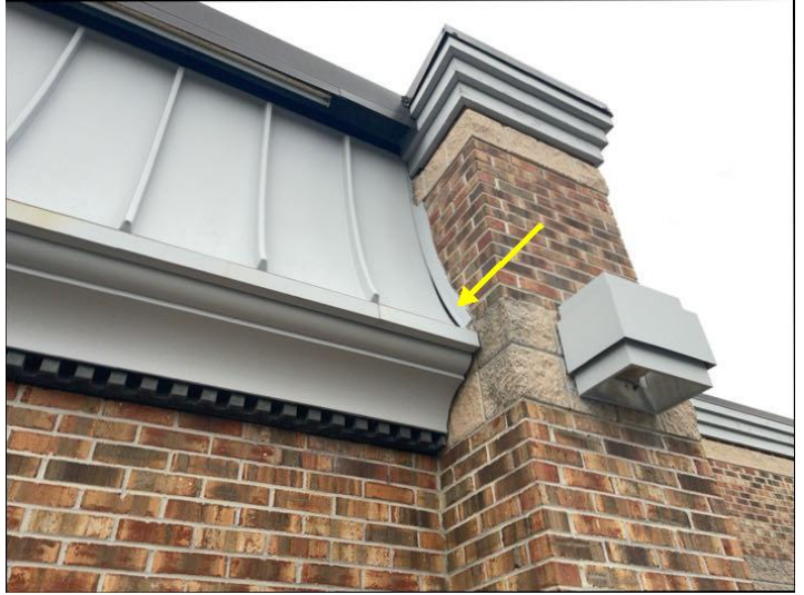
Loose flashing
