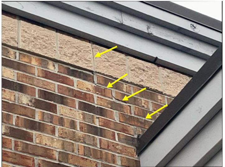
Step crack
