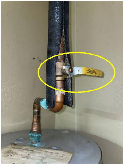
Water shut off valve
