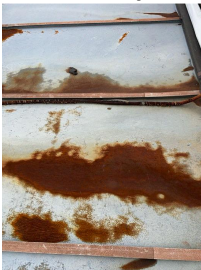
Corroded roofing
