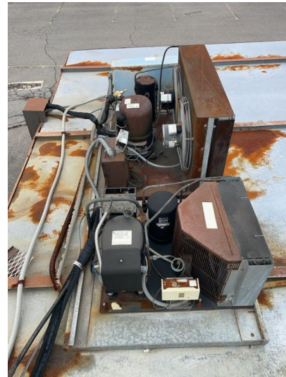
Compressor cover missing
