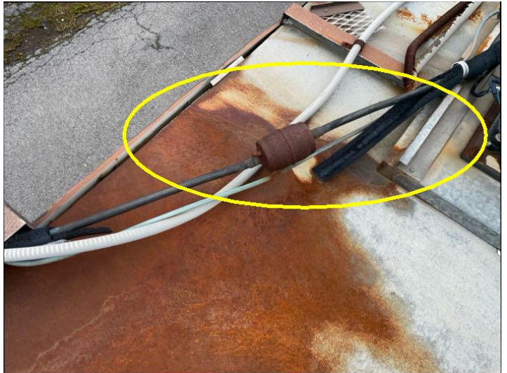
Deteriorated insulation
