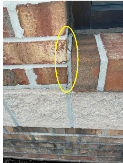
Deteriorated mortar
