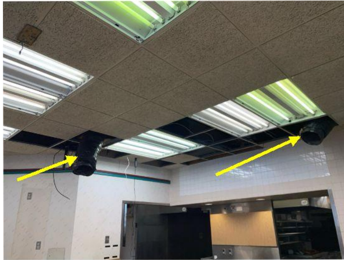
Register vents missing
