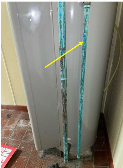
Overflow discharge pipe
