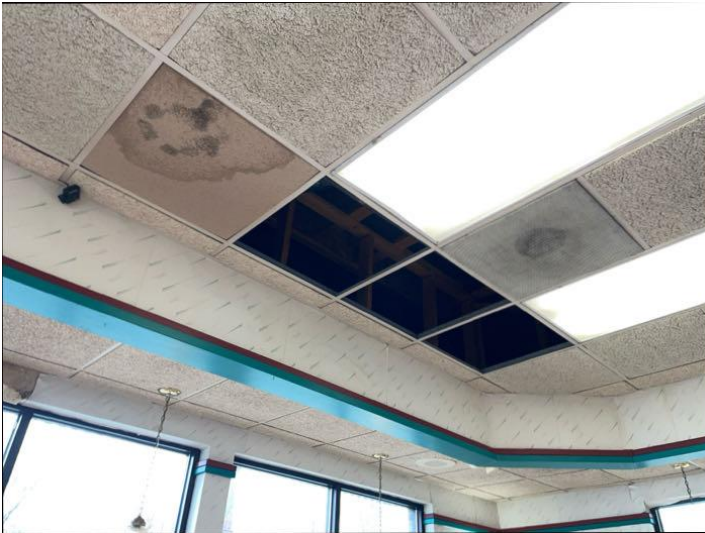
Stained and missing tile
