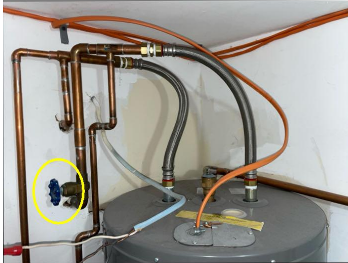
Water shut off valve
