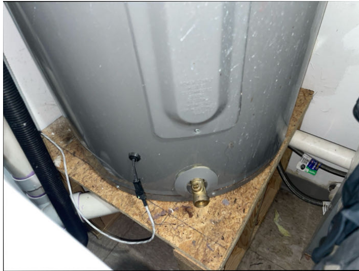
Overflow pan and drain missing
