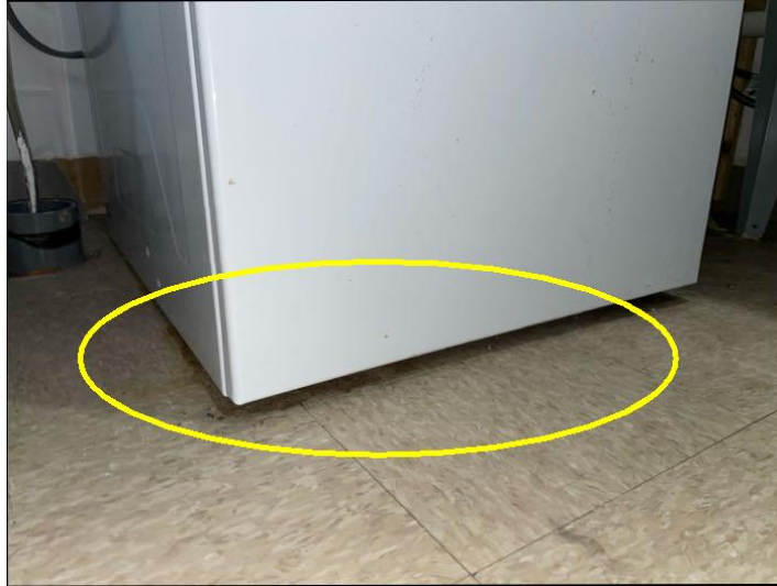
Overflow pan missing
