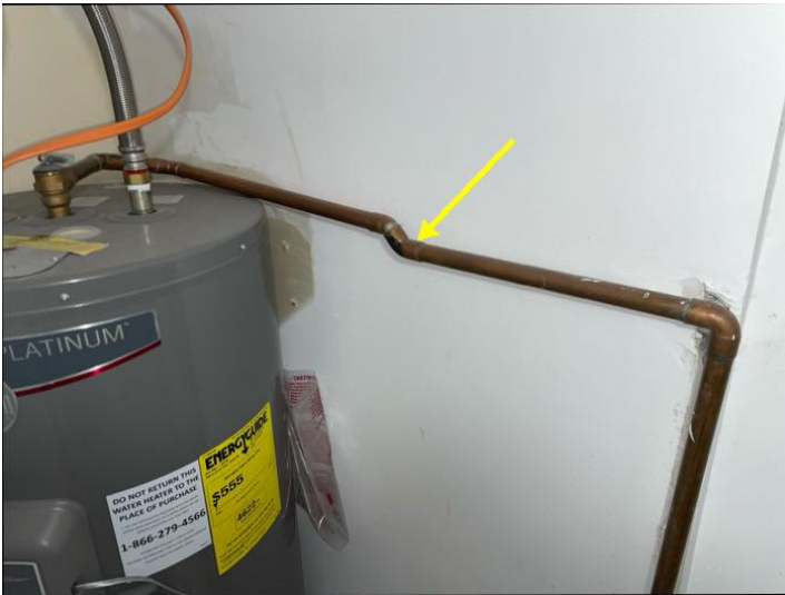
Overflow discharge pipe
