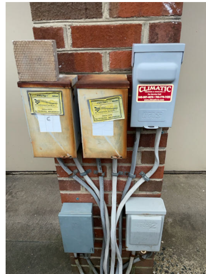
Unmarked disconnect boxes
