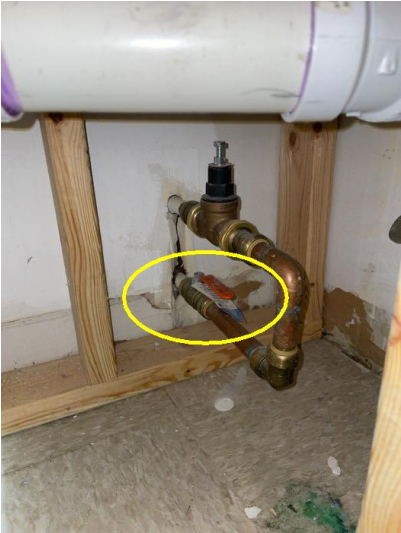
Main water shut off valve
