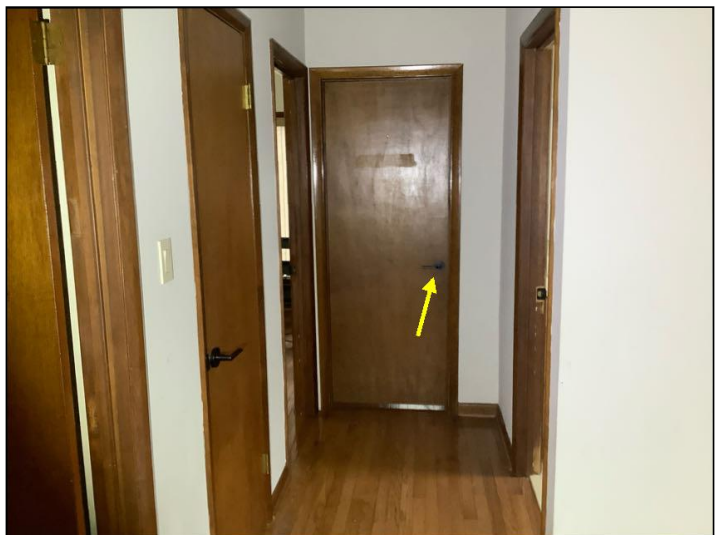
Closet door locked at the time of the inspection
