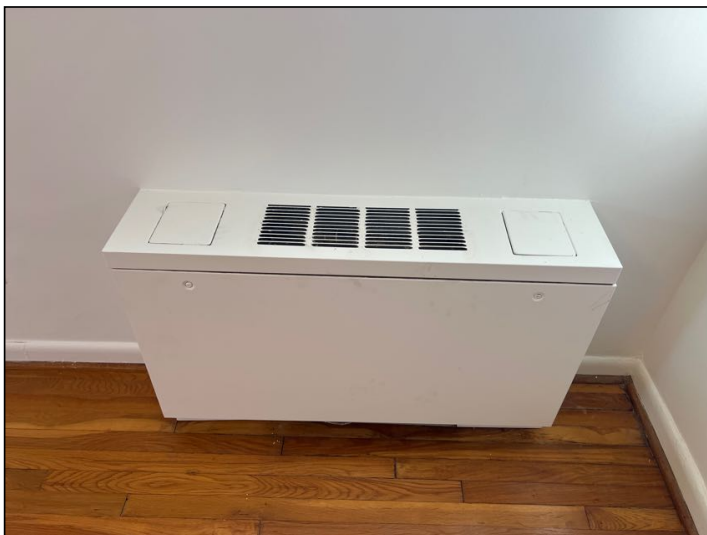
PTAC (fan coil)
