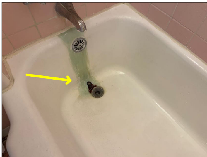
Discoloration/corrosion
