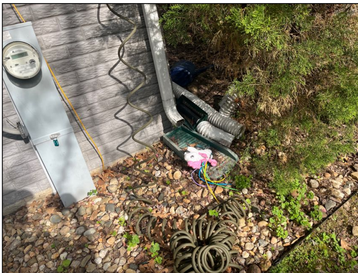
Terminates near foundation
