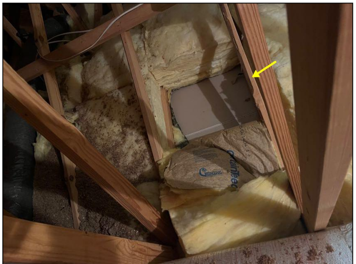
Missing/loose insulation
